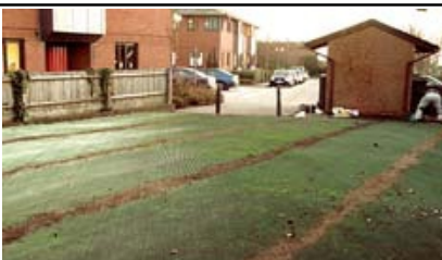
Mesh upon installation
